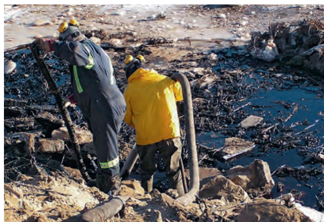
Figure VI-2.2D Vacuum system to recover oil on ice surface (Source: ECRC).
