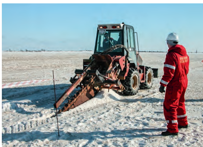
Figure VI-1.3B Ice trenching across the intertidal zone (Photo credit: E. Owens).
