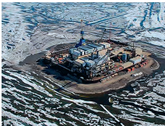
Figure C.6 Northstar oil production island in shallow water (12 m) off Prudhoe Bay (Photo: Lori Murray).
