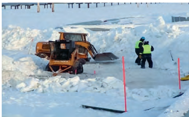
Figure VI-1.3D Snow removal on tundra to detect subsurface oil in snow (Source: Alaska Clean Seas).
