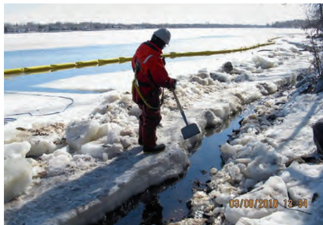
Figure VI-2.2B Trench cut in ice to collect oil for recovery (Source: ECRC).
