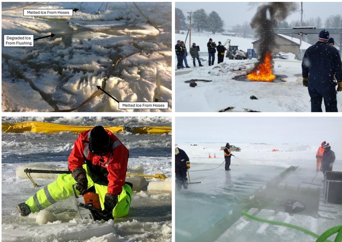
Figure 3-4. Ice degradation can come from many sources in the response including warm hoses, burning operations, flushing, and cutting ice for containment and recovery. Photos: ACS.
