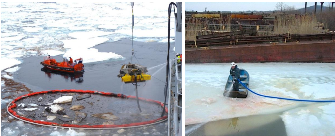
Figure 6-29. (Left) Skimmer being flushed clean over oil and ice in a containment boom. This is the same procedure that could be used flush ice blocks. Photo: T&T. (Right) Flushing contaminated ice surface from small boat. Photo: D. Dickens.
