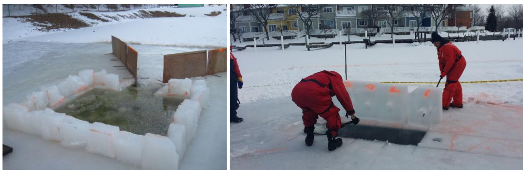
Figure 6-22. (Left) Ice berm built around a recovery sump with plywood barriers funneling oil under ice into the sump. Photo: ACS. (Right) Ice blocks being removed from a slot and placed along the edge to create a berm. Photo: Enbridge.
