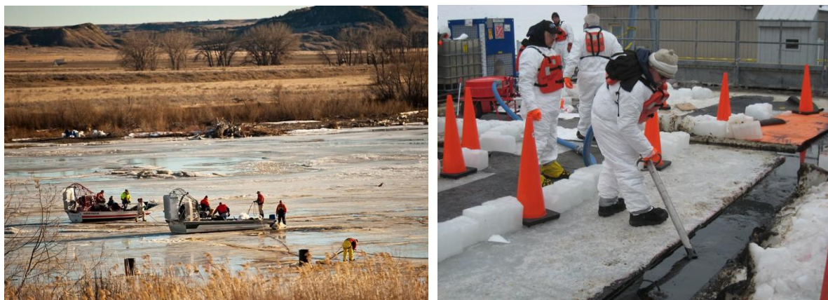
Figure 6-27. (Left) Recovery of oil on thin ice using vacuum systems from airboats on the Yellowstone River. Photo: Enbridge. (Right) Recovery of oil from a trench using direct suction with a peristaltic pump. Photo: ACS.
