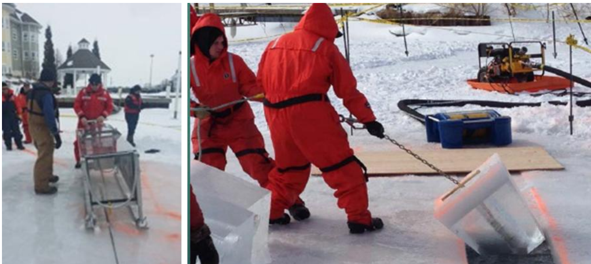
Figure 6-17. (Left) A horizontal chainsaw sled designed to cut blocks at an angle, creating a wedge shape for easier removal. (Right) An ice block being pulled from a slot after cutting. Photos: Enbridge.
