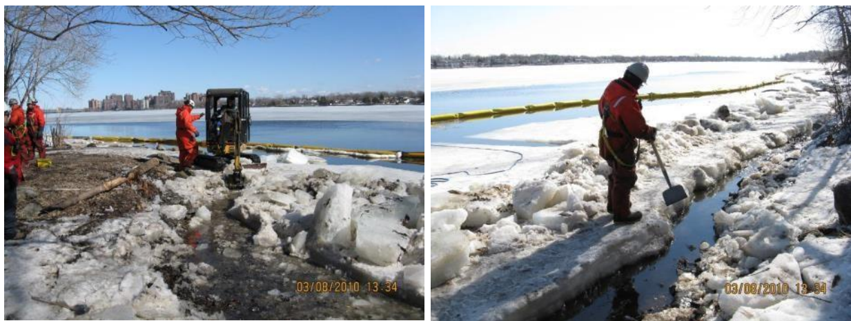
Figure 6-14. Trenching on shoreline with excavator. Photos: Enbridge.
