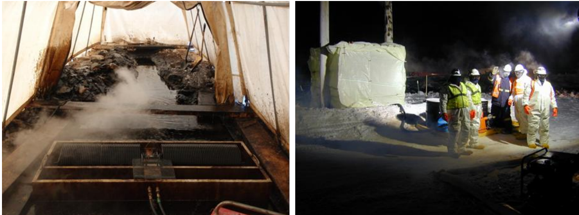
Figure 6-8. (Left) Example of small, heated shelter erected over a recovery hole to keep personnel and equipment warm. Photo: ACS. (Right) Reinforced plastic sheeting built around scaffold and held with spring clamps. Photo: Enbridge.
