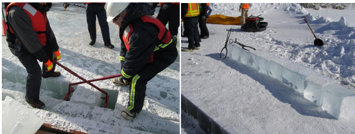
Figure 6-21. One- and two-person ice tongs are used to lift small- and medium-sized blocks from the trench. Photos: ACS.
