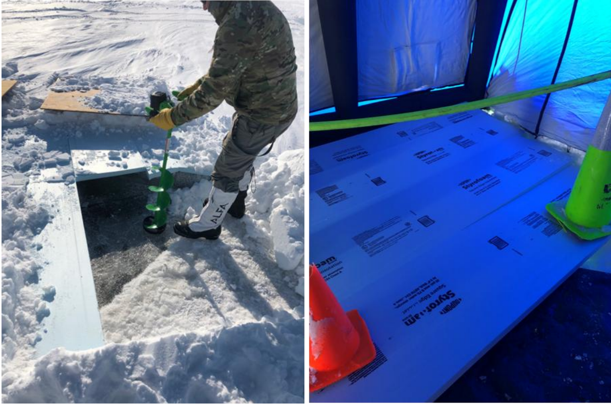
Figure 6-10. Insulating openings. (Left) Blueboard foam placed over opening and covered in snow outdoors. (Right) Blueboard foam covers opening in a shelter. Photos: ACS.
