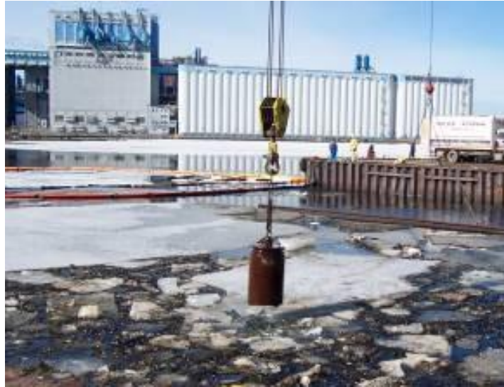
Figure 6-3. Heavy steel weight breaking oiled ice in Thunder Bay. Photo: ECRC.
